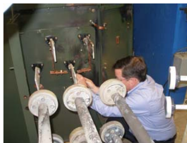
Jim, in the high power lab setting up an arc flash test on a pad mount transformer.
