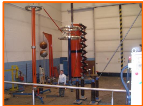
A side trip to the high power lab during an IEC meeting in Frankfurt Germany.
